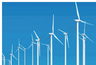
Wind Power Generation
